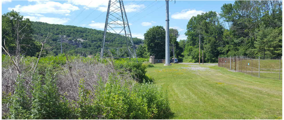
Invasive plant species may overtake utility structures and require removal.
